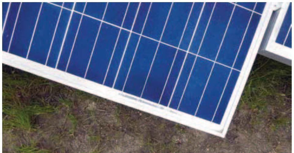
A downward-pointing corner prevents dirt collecting along the frame, and the residue at the bottom corner is reported to be significantly less.
